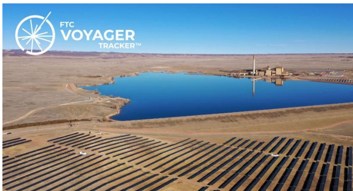
EPC Contractor Colorado – 29 MW
